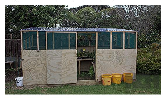
With the help of a brother who just happens to be a builder we settled on a kitset type design. The four walls were prefabricated and assembled onsite with the roof being fitted to tie it all together. Pavers yet to be installed over the floor area.
